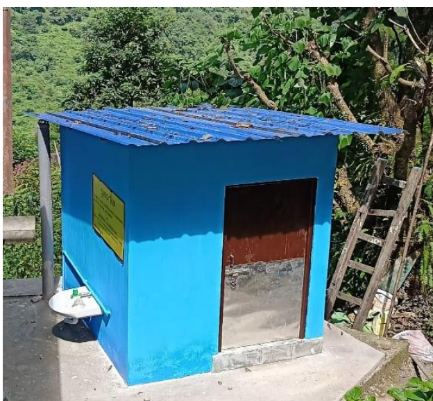
Construction of community toilet at Lingdok, East Sikkim
