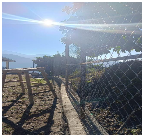
Construction of fencing/ barricading works at School, North Sikkim
